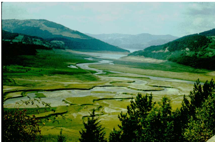
Fig. 11. Izvoru Muntelei Reservoir. View on upstream sedimentation area after a period of emersion.
